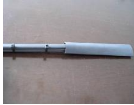
27. Shrink the tube completely. Start at end farthest from the cap and work toward the open end. Keep heating after tube has shrunk, to melt adhesive and mastic inside tube. Total heating time should be about 5 minutes (Temperature about 400°C(752°F))
