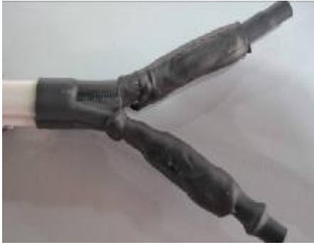
25. Squeeze the mastic together
