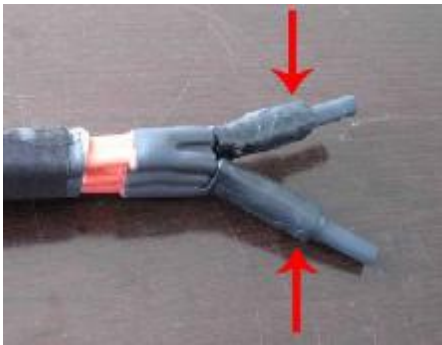
25. Squeeze the mastic together
